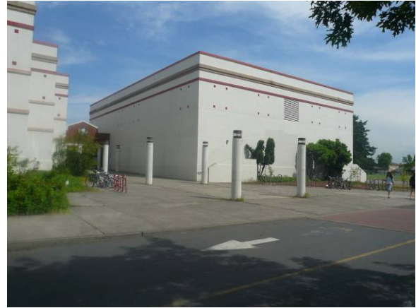
North elevation facing south
