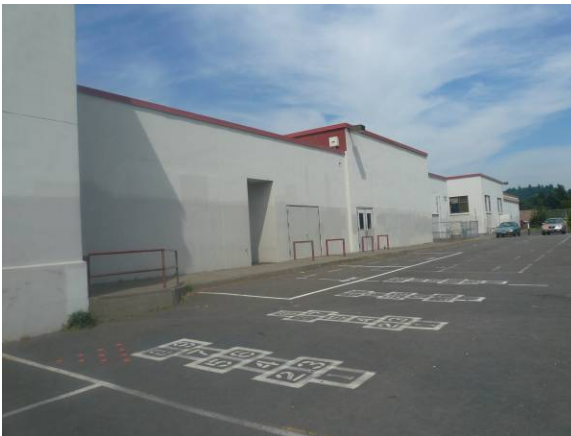
West elevation facing east
