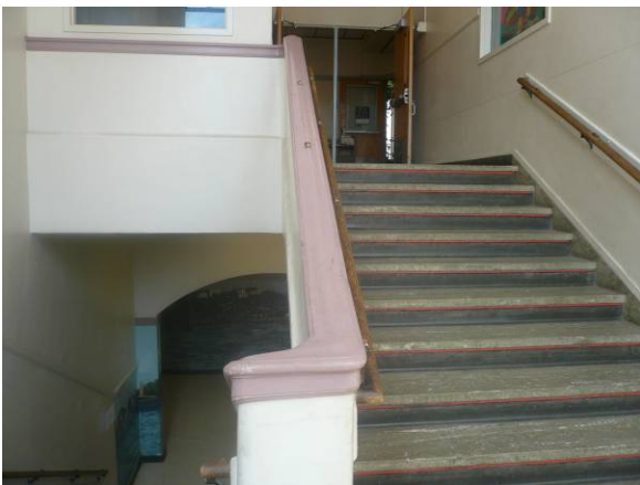
Staircase with handrail
