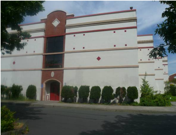
North elevation facing south
